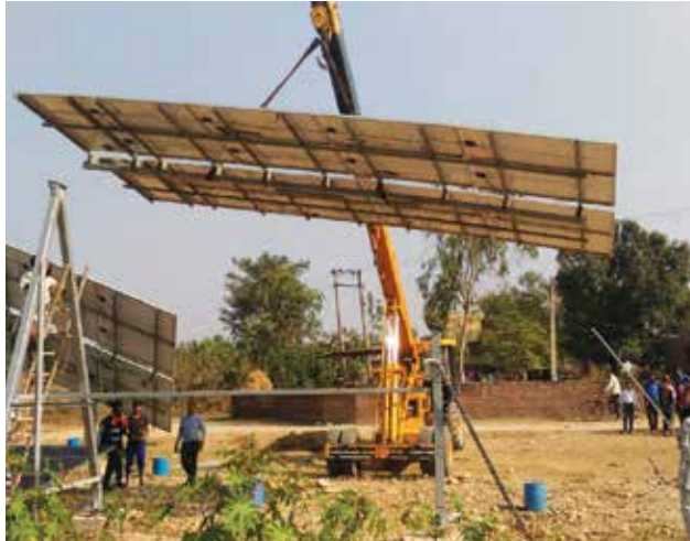
Solar Tracker Installation
