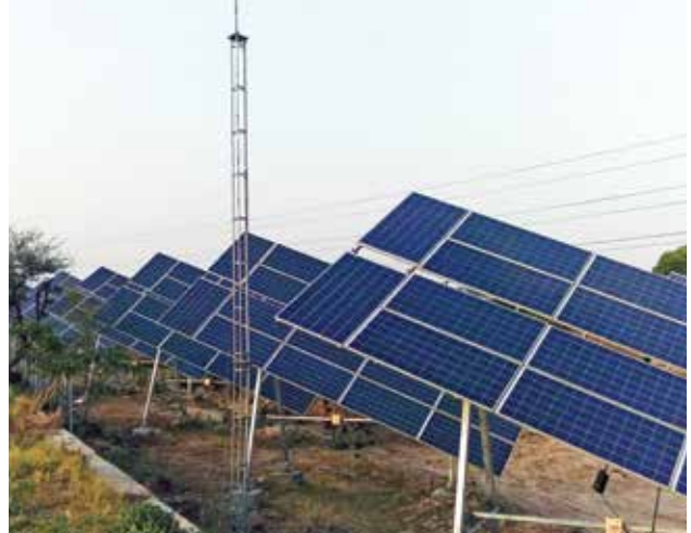
Solar Trackers Installation
